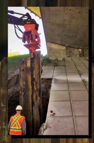
Simple operation means that any excavator operator can easily drive and extract piles
